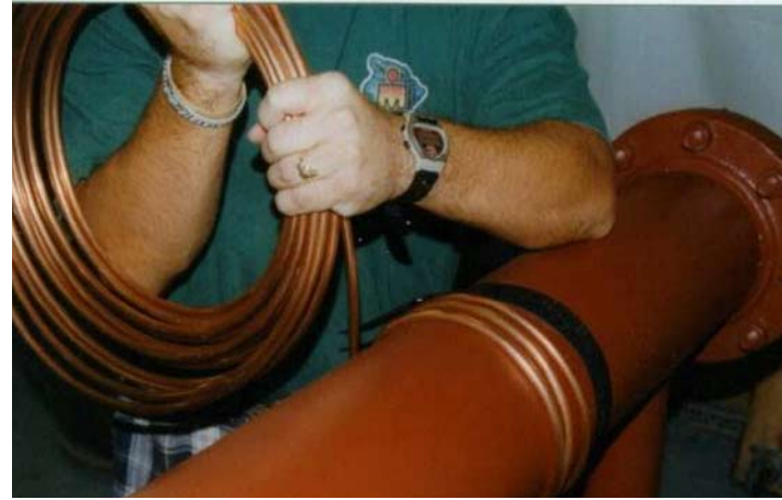
Wrapping a 6-inch pipe with copper tubing.
