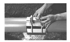
Loosely close the clamp around the pipe by lifting the C-Plate lip over the lug system stainless receiver bar, meeting the stud and fingers, and lock in place. Rotate the clamp slightly in the direction of the arrow stamped on the clamp band to ensure the tapered gasket lies flat under the clamp.
