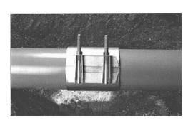
5/8" Bolts/Studs tighten to 70 Foot Pounds of Torque\*
