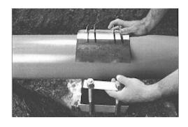
Open the repair clamp by loosening (without removing) the nuts to the top of the stainless studs/bolts. Disengage the locking "C-Plate" and lift plate to open clamp.
