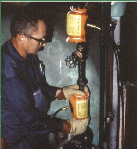
QWIK-FREEZER™ IS USED TO MAKE A DOUBLE FREEZE ON A PIPE IN ORDER TO ISOLATE A VALVE.
