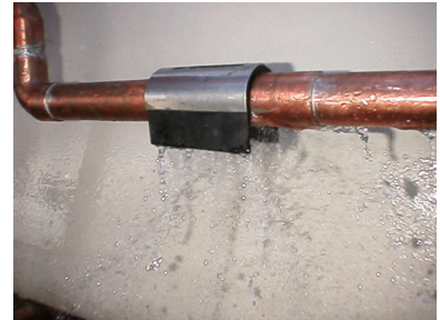
Loosen the bolt and separate the two parts of the clamp. Snap top half of clamp with rubber directly over leak
